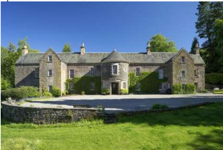
Figure 2 – Foswell House, Auchterarder, home of the world's first domestic heat pump
